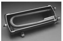
cause of the small hole drilled in the bottom bend of this tube liquid refrigerant will also collect here. On start-up liquid refrigerant could then be sucked out of the tube and return to the compressor. To prevent this from occurring, a small hole is drilled at the top end of the tube. This small hole equalizes the pressure on both sides of the liquid in the tube and prevents the liquid refrigerant from being sucked out on start-up.
